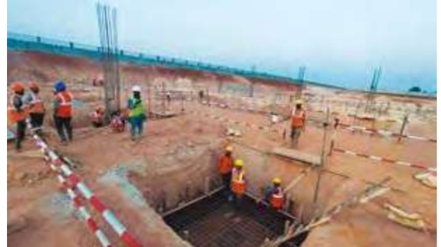
▶ On the ground, construction activity has been initiated
