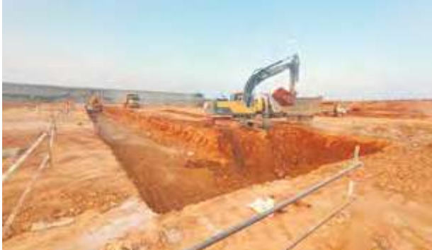
▶ Site-enabling work has been completed
